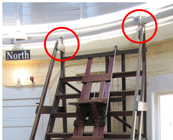
Avoid positioning the observer's chair directly under the dome drive cable rail. There are places where the chair and the rail make contact.
